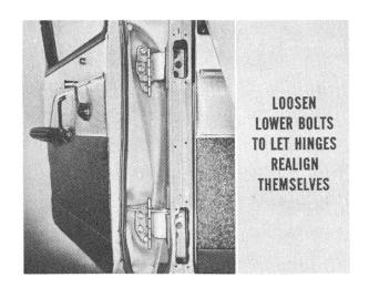
Then, retighten the bolts. A straight hinge-pin line is important, or you'll end up with a heavy-dragging door. It will help to swing the door a few times to be sure you've eliminated any bind caused by the hinge pins being cocked.
